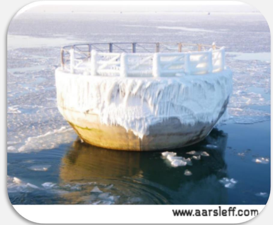
Picture borrowed from Aarsleff. Showing sea ice on a Gravity Based Foundations.
